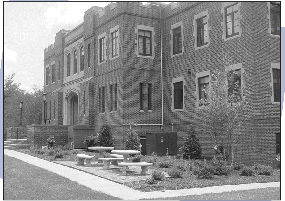
Completed landscaping outside the Shuford Science Building
