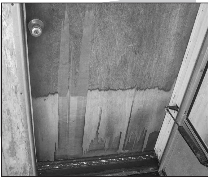
Water damage on front door of Douglas home
