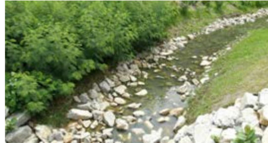
Bioswale Channels
