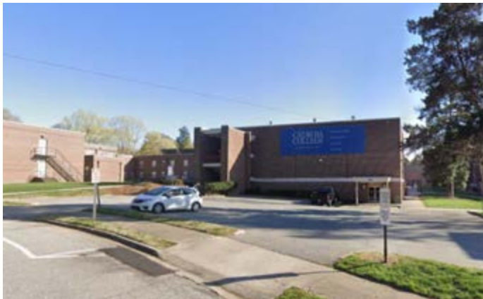
Existing conditions – P10 Hoke Hall Parking
