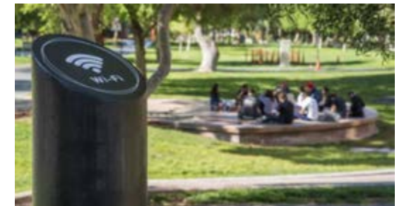
Wi-Fi & Electrical Infrastructure
