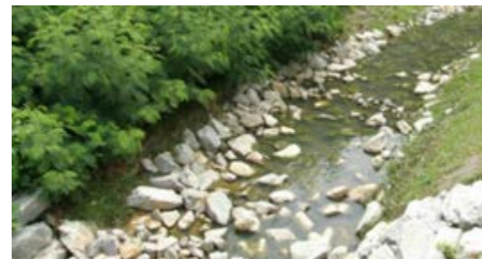
Bioswale Channels
