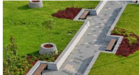
Permeable Pavement
