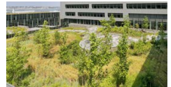
Intensive Green Roofs
