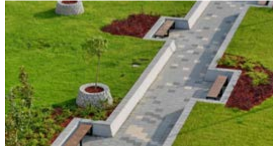
Permeable Pavement
